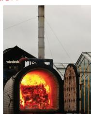
fuel. The batch-loaded boilers predominantly use straw but, of course, the area of the country has a bearing on the selection of the fuel source. Boilers that run on wood chips/pellets or straw pellets have automatic feeding systems from a hopper on the side of the boiler.
